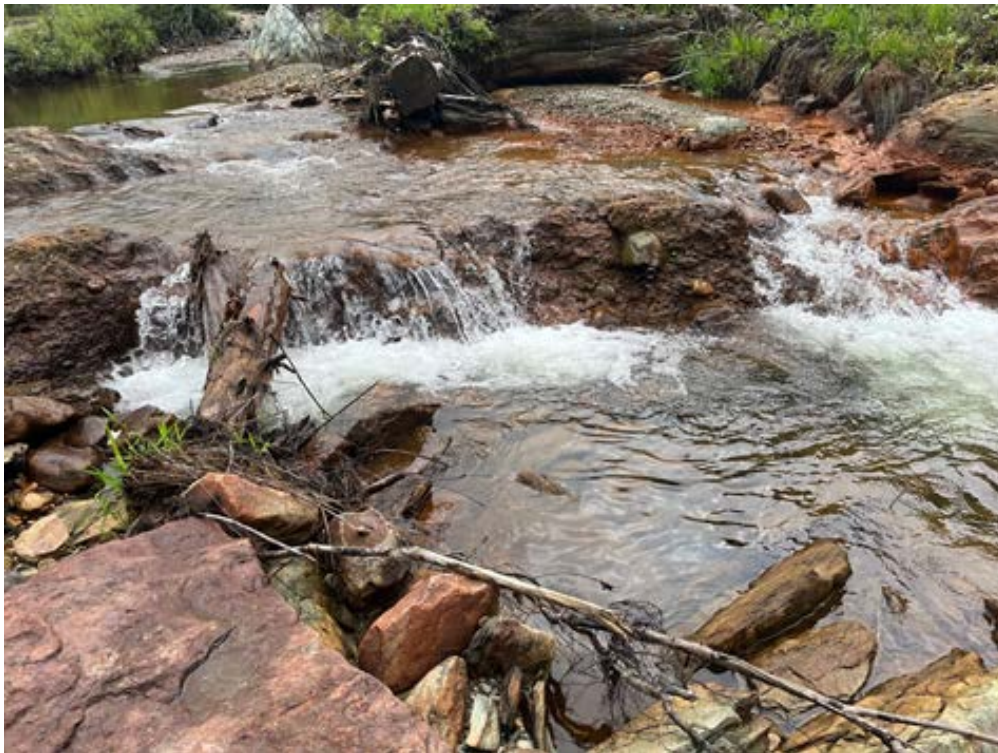
Figure 5. Looking upstream at remaining concrete uncovered during Year 2 monitoring.
